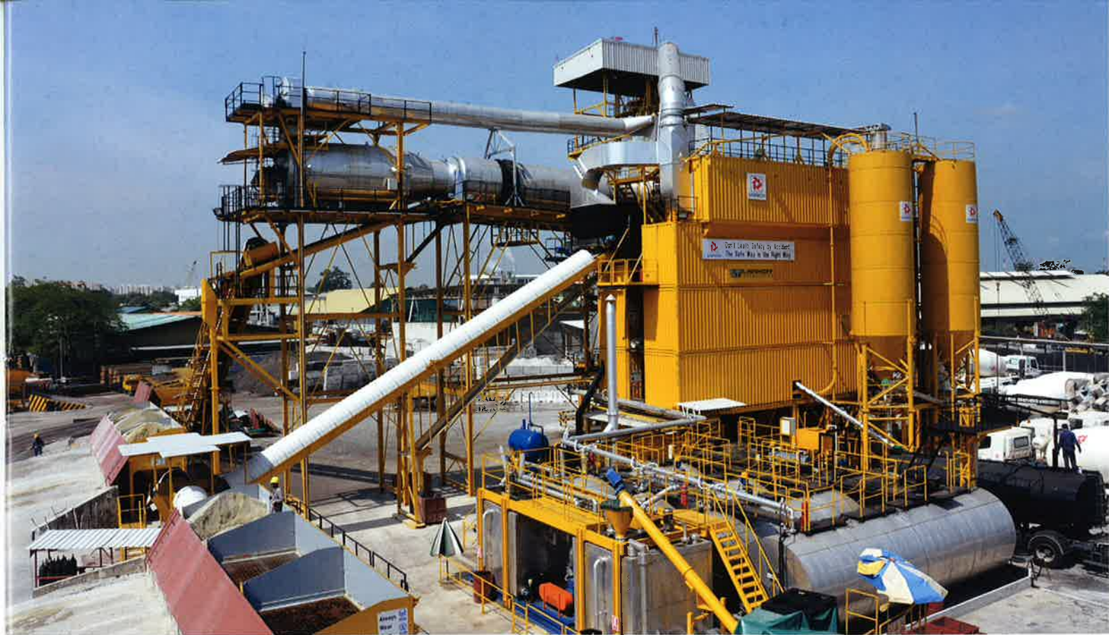
Asphalt recycling plant.
