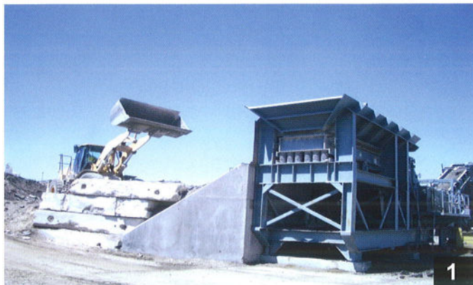
1 Loading of asphalt pavement waste for crushing
