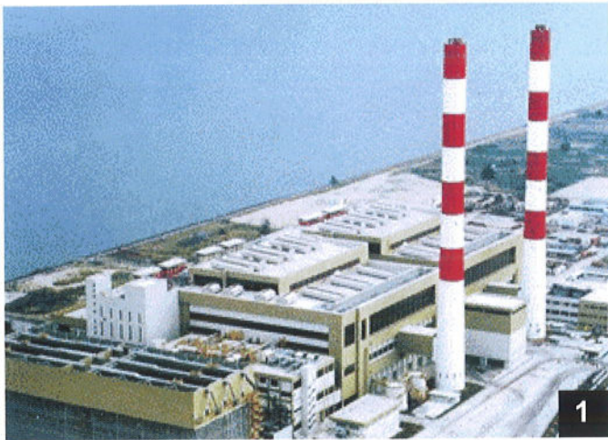
IBA is produced after the incineration process
