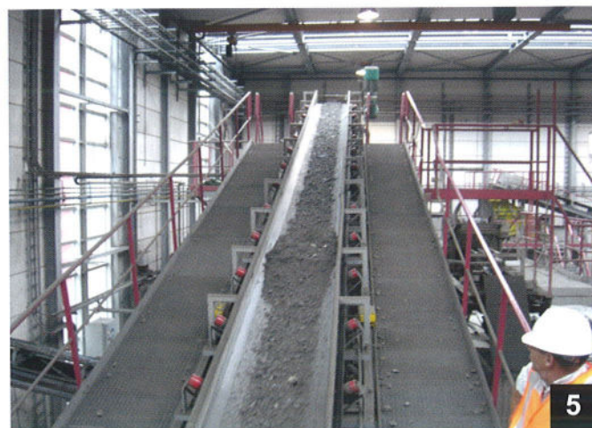
Chemical treatment of IBA using a patented system
