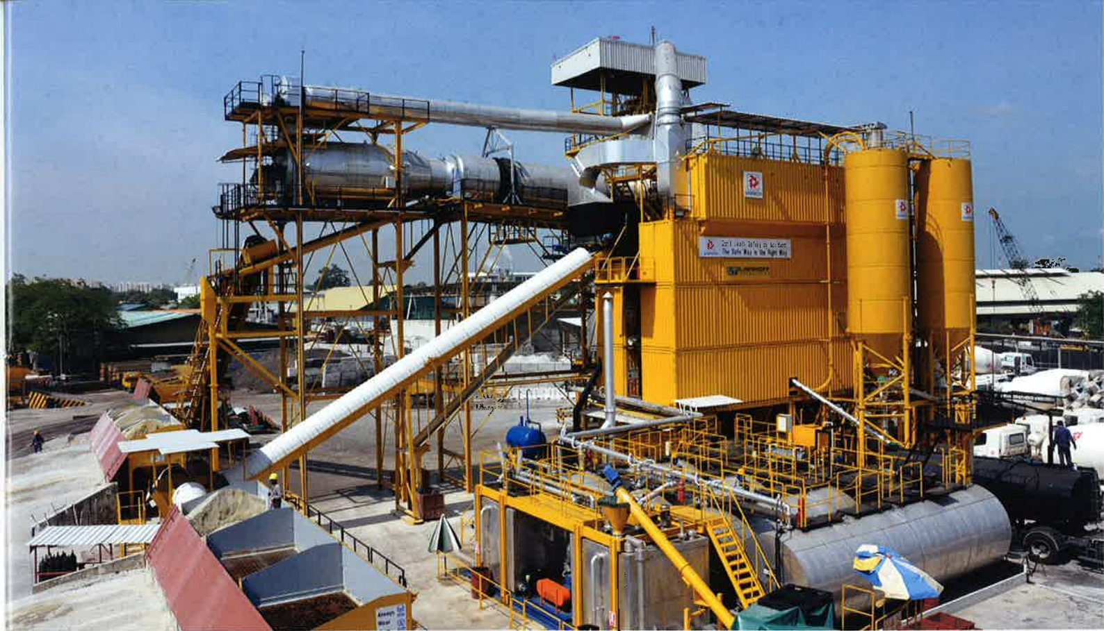
Asphalt recycling plant.
