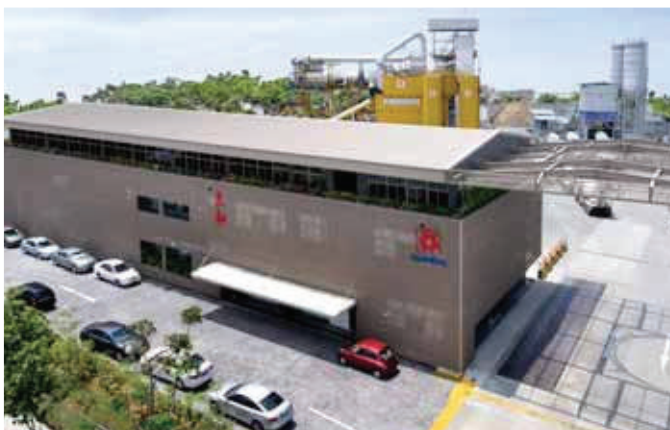
Aerial view of Samwoh Eco-Green Park
