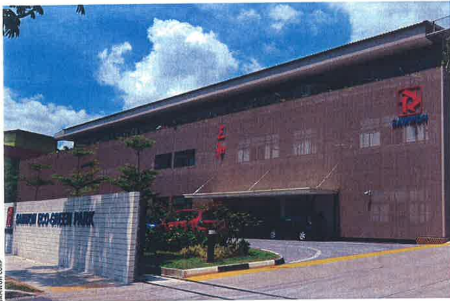
The Samwoh Eco-Green Building. Ho's pride and joy, is the first building in the region to use concrete with up to 100% RCA and was awarded the BCA Green Mark Platinum Award
