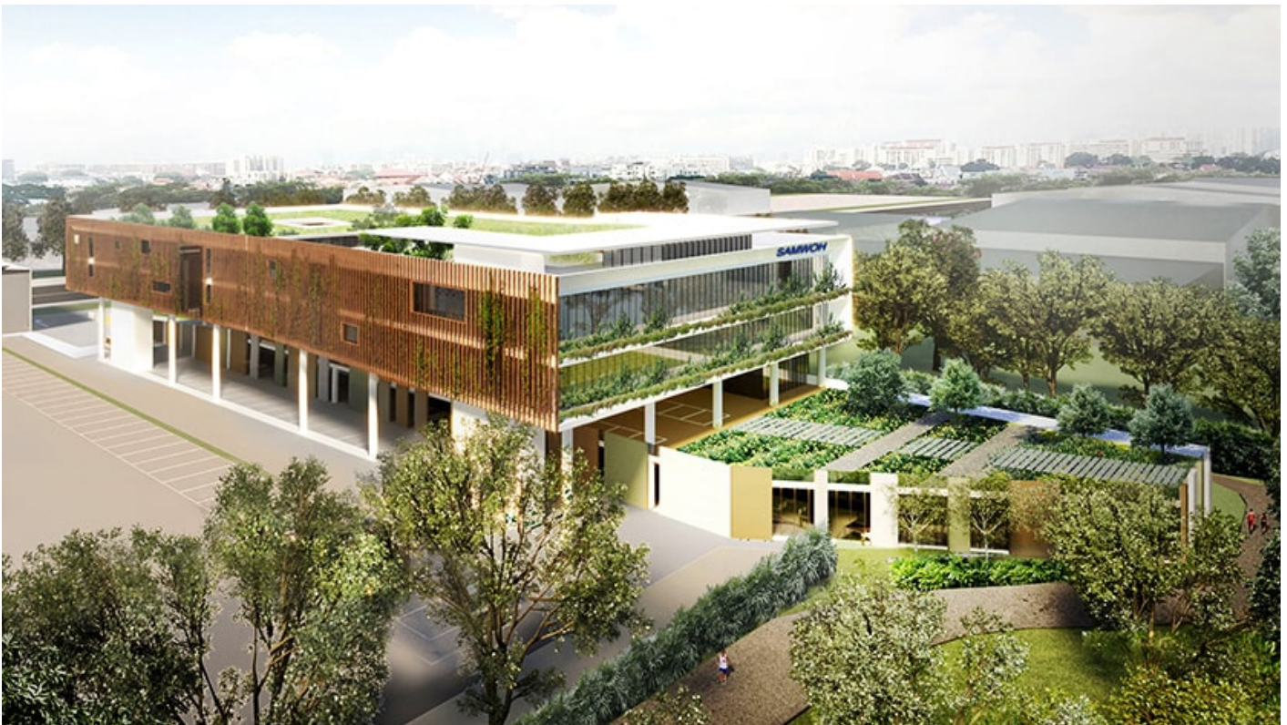
Samwoh Smart Hub will be the first positive energy industrial building in Singapore (Photo credit: Samwoh)
